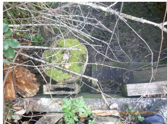
Figure 15.3 West abutment - Rotting and hollow backing plank spacer.
