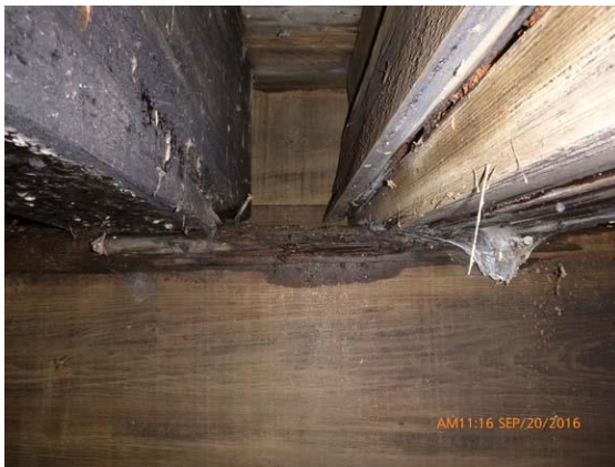
Figure 3.1 Pile cap - The cap is rotting and starting to crush under the center stringers of the west abutment. Also note the longitudinal splits and decay on the stringers.
