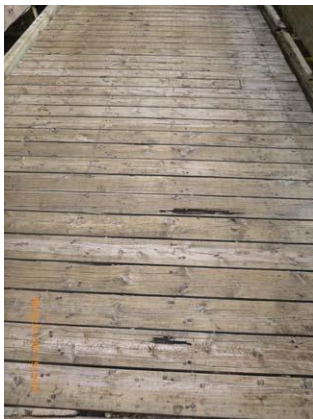
Figure 5.1 Deck - Moderate deterioration throughout and patches.
