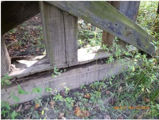
Figure 1.13 Pier 9 - Rot and severe section loss of bottom pile cap.
