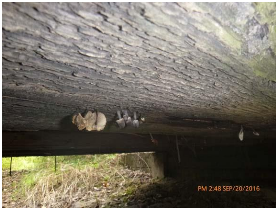
Figure 8.1 Beam - Deterioration and section loss of north stringer.
