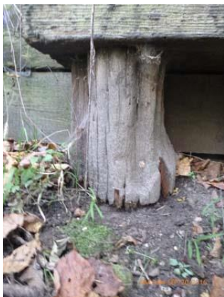
Figure 1.3 East Abutment - Rotting and splitting pile with section loss at ground line.
