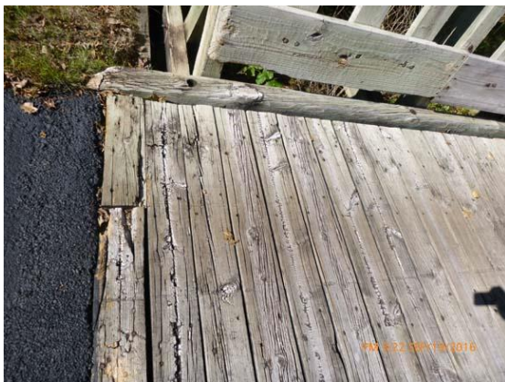
Figure 17.1 Deck - Planks rotting towards the end of deck.
