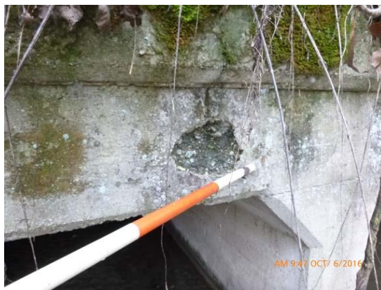
Figure 18.4 North Head Wall - Moderate spall over center barrel.
