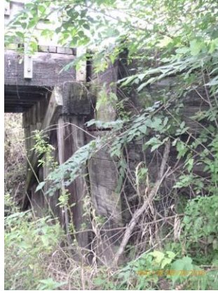
Figure 3.4 East abutment - Rotation of the backing planks.
