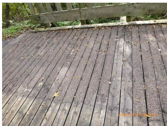
Figure 12.2 Deck - Overlay experiment with some material loss.
