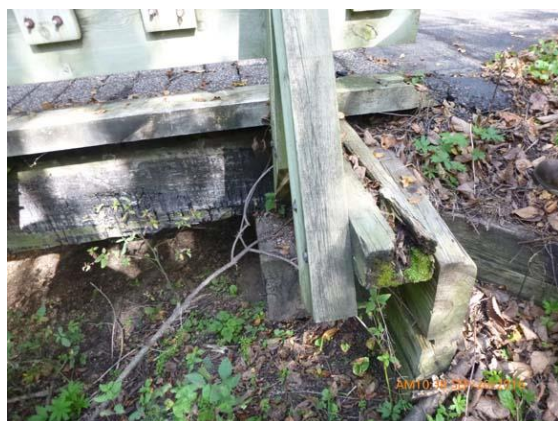
Figure 12.3 Deck - Floor beam at southeast corner rotting.
