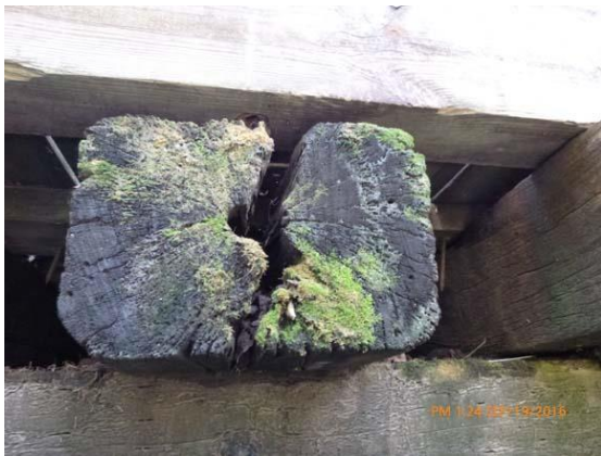
Figure 16.1 Floor beam - Typical floor beam failure due to rot.
