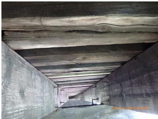
Figure 9.1 Floor beams - Typical floor beam failure due to rot.
