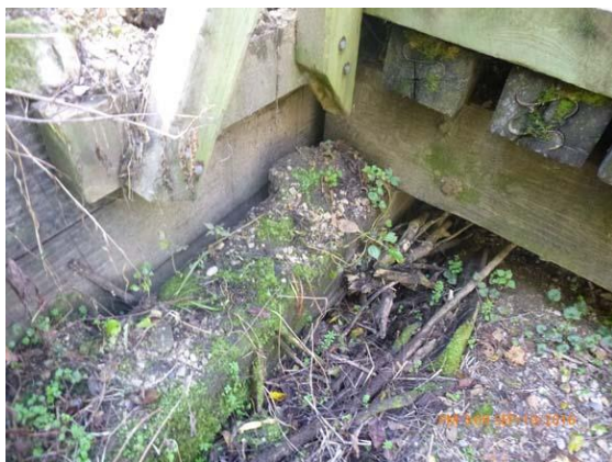
Figure 6.2 West abutment - Cap partially buried and starting to decay.
