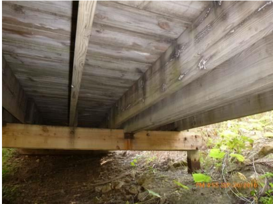
Figure 19.1 Beams - Minor weathering throughout. Note the staining due to rusting of the beam brackets.
