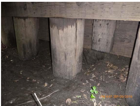
Figure 14.3 East abutment - Minor undermining under backing planks.
