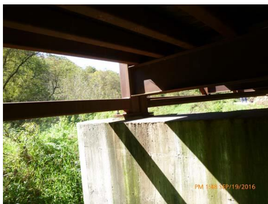
Figure 11.4 Pier bearing - Grout in good condition.
