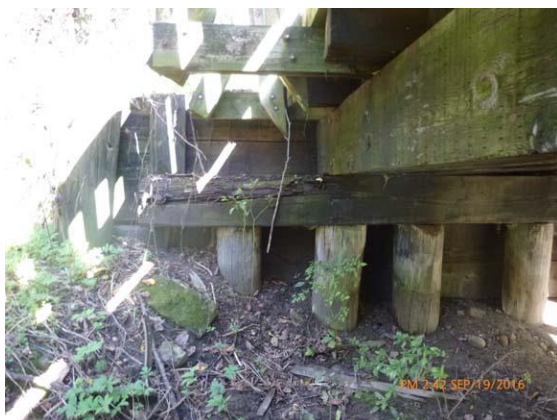
Figure 9.2 East abutment - Cap splitting and decaying.
