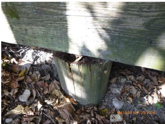
Figure 1.2 West Abutment - South pile rotting and becoming hollow.
