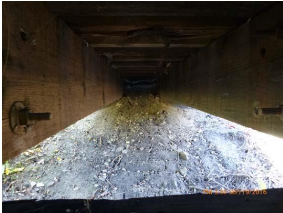
Figure 17.3 East abutment - Piles are completely buried and cap is partially buried.
