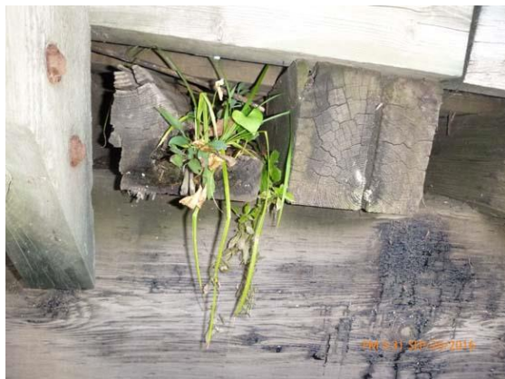
Figure 13.2 Floor beams - Typical floor beam failure due to rot.
