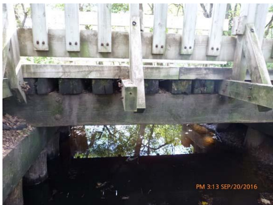
Figure 4.2 Deck - Floor beams failing and splitting.
