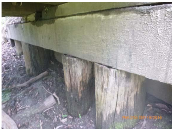
Figure 5.4 East abutment - Rotting and splitting piles becoming hollow.
