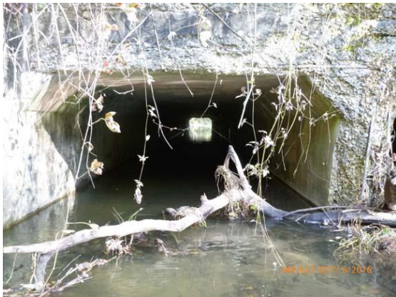
Figure 18.1 South Head Wall - Extensive damage to headwall with exposed rebar, and spalling of the barrel ceiling.
