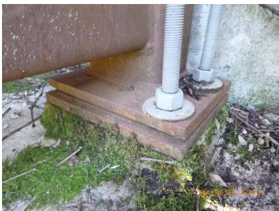
Figure 11.3 Southeast bearing - Grout with minor deterioration.
