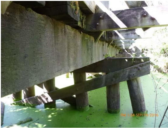
Figure 16.3 Looking West - Piers and beams in good condition. Note the generalized failure of the floor beams.
