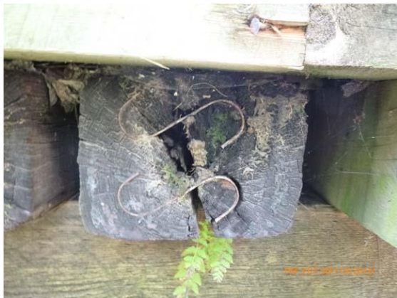
Figure 6.1 Floor beams - Typical floor beam failure due to rot.
