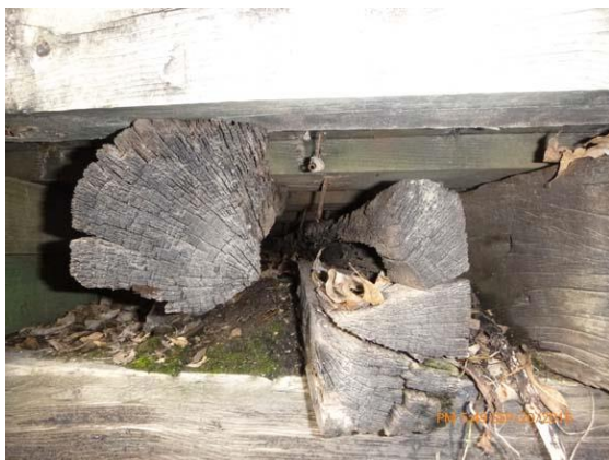
Figure 7.2 Floor beams - Typical floor beam failure due to rot.
