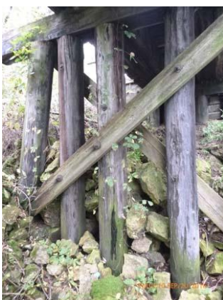
Figure 2.6 Pier 1 - Rocks stacked against piles and cross braces.
