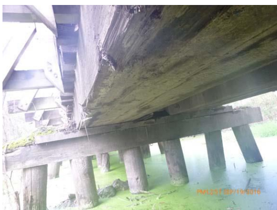
Figure 5.6 Pier 4 - Bearing spacers shifting. Note minor impact damage on fascia stringer.
