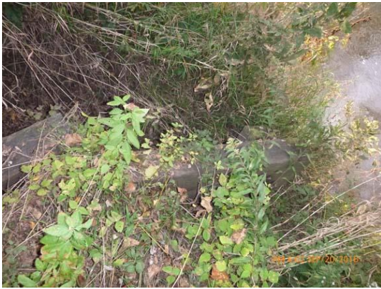
Figure 14.5 Northeast wingwall - the wall is rotating forward and failing.
