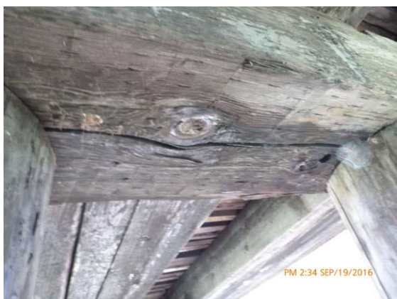
Figure 9.5 Pier 3 - Major splitting of the pile cap.
