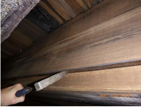
Figure 3.3 Beams - Longitudinal splits and decay on beams.
