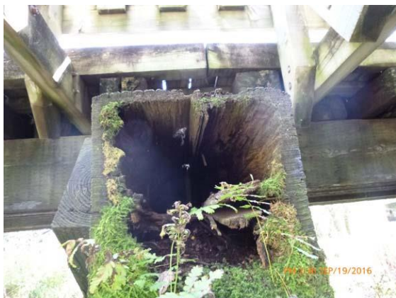
Figure 9.4 Pier 2 - Major decay and section loss on pile cap.
