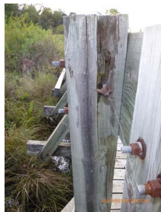
Figure 13.3 Rail - Deterioration of the rail posts at the south side.
