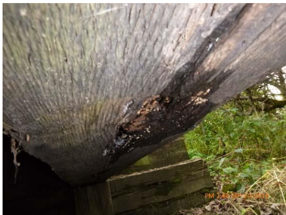
Figure 8.2 Beam - Deterioration and section loss of north stringer.
