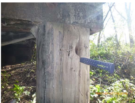
Figure 12.6 Piles - South pile of the east pier becoming hollow and rotting.
