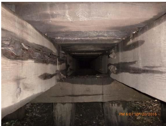
Figure 14.2 Beams - Minor decay along the inside of interior stringers.
