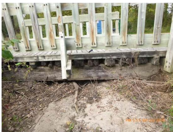
Figure 7.3 Looking north - Buried abutments and failed floor beams.
