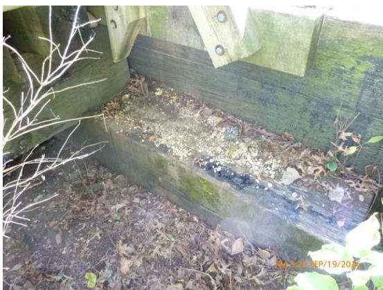
Figure 17.2 West abutment - Piles and cap are partially buried.
