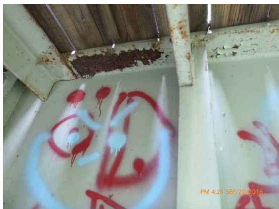
Figure 20.3 Beam - Typical localized paint system failure.
