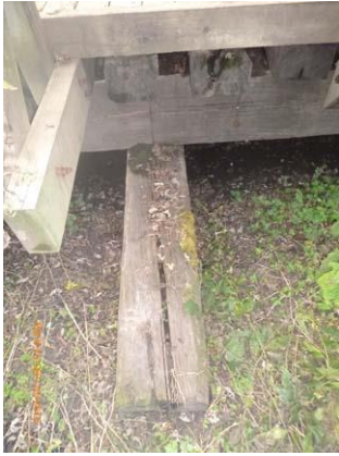
Figure 14.4 Pier cap - Moderate split at pile cap.
