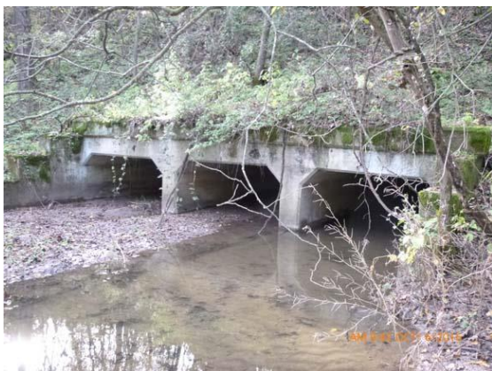
Figure 18.3 North Head Wall - Headwall in good condition.
