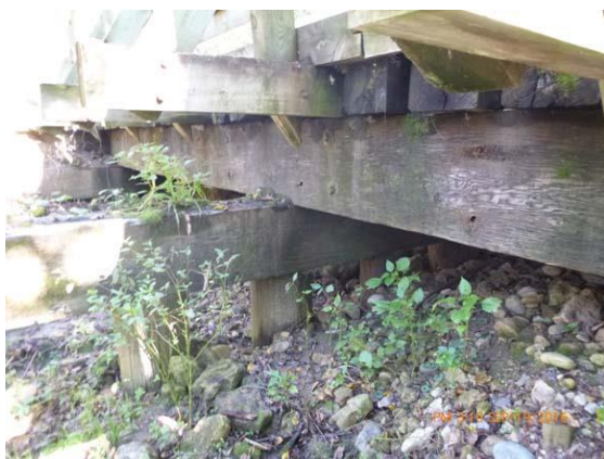
Figure 6.3 Pier - Cap decaying and rotting, and piles becoming hollow.
