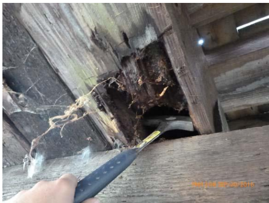
Figure 2.2 Beams - Section loss and rot at bearing areas.
