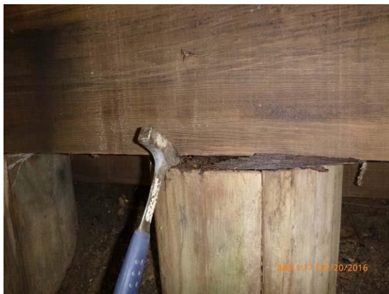
Figure 3.2 Piles - On the west abutment piles are rotting and splitting.
