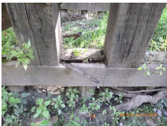
Figure 1.11 Pier 7 - Rot and significant section loss of bottom pile cap.
