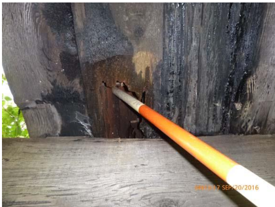
Figure 1.9 Pier 7 - Beam section loss and rot at bearing.
