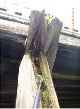
Figure 3.6 Pier 2 - North portion of pile cap and north pile have severe decay and have failed.
