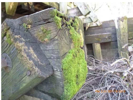
Figure 9.3 Pier 1 - Decay on pile cap ends.
