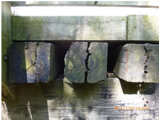
Figure 10.1 Floor beams - Typical floor beam failure due to rot.
