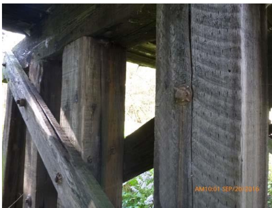
Figure 1.8 Pier 6 - Most columns and bracing are splitting.
