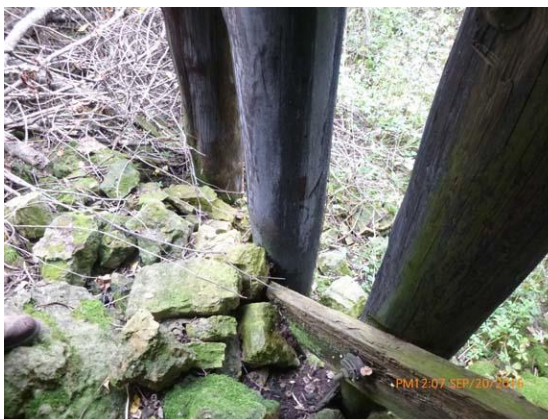
Figure 2.5 Pier 1 - Rip-rap crushing ends of cross bracing.
