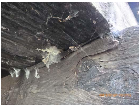
Figure 1.14 Pier 9 - Local crushing of the pier cap under beam.
