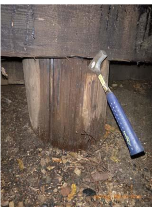
Figure 12.7 Piles - West abutment center piles are becoming hollow and rotting.
