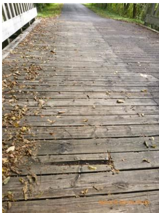
Figure 12.1 Deck - Minor deck plank splitting.
