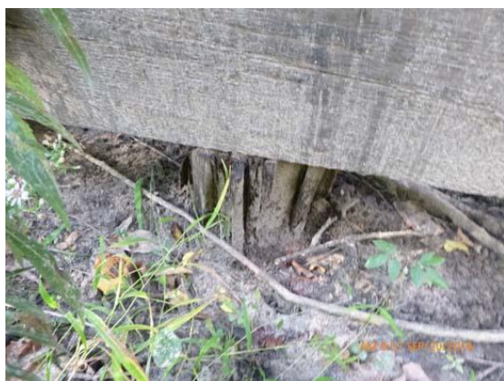
Figure 1.10 Pier 7 - Pile rotting through.
