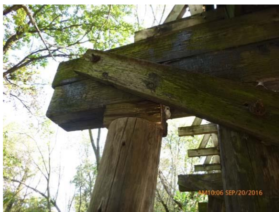
Figure 1.6 Pier 2 - Wood block installed to fill the gap between top of pile and cap.
