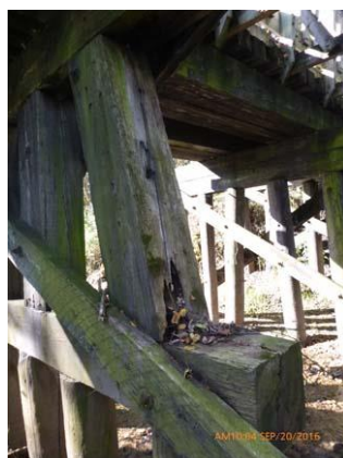
Figure 1.7 Pier 3 - Severe section loss and splitting of the north column.
