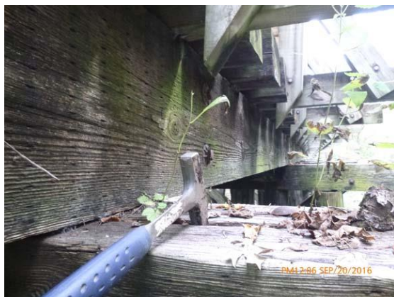
Figure 2.3 Piers - Splitting and decay of pile caps.
