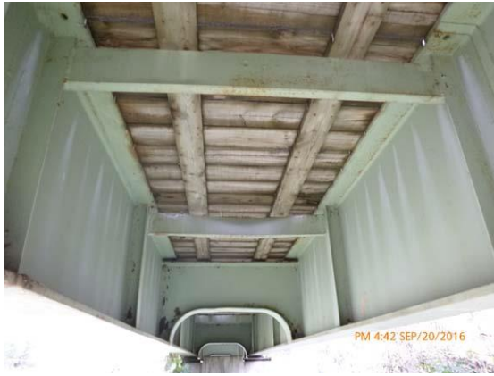
Figure 20.4 Diaphragms - Note the slight bending of the diaphragm at the center of the picture.
