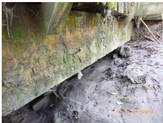
Figure 10.2 Beam - Active moss on beam. Note the buried footing.
