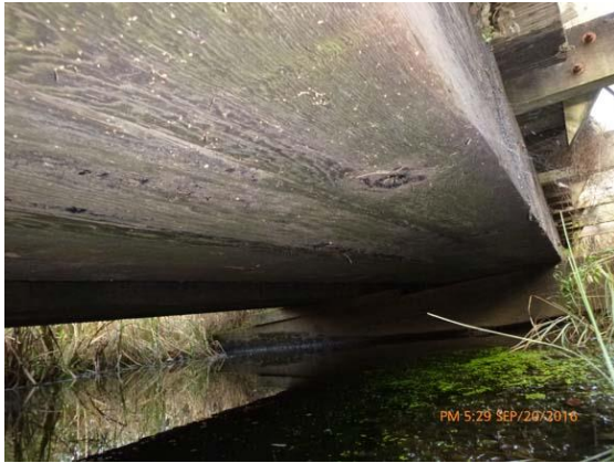
Figure 13.4 Beams - Beams in good condition. Note how the north beam bearing spacer has shifted slightly at Pier 2.
