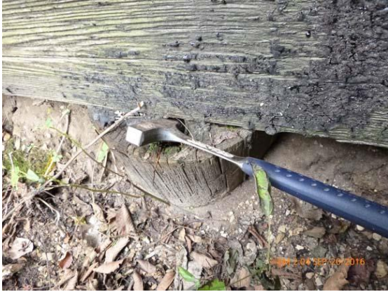
Figure 15.4 East abutment - Top of pile rotting and becoming hollow.
