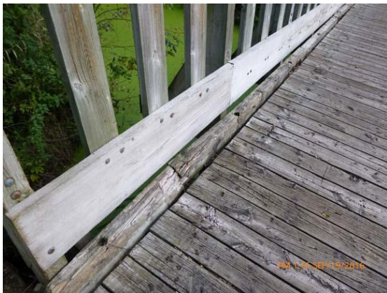
Figure 16.2 Deck - Decaying curb sections.
