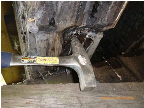
Figure 12.5 Stringers - Minor section loss at pier bearing.
