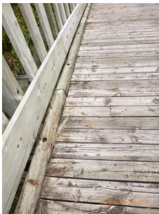
Figure 15.1 Deck - Damage to curb section.
