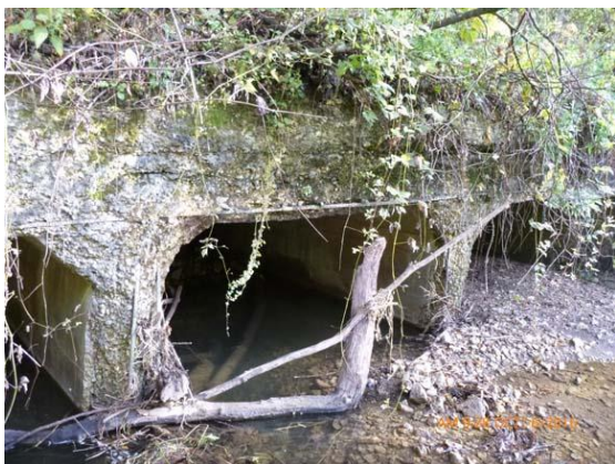
Figure 18.2 South Head Wall - Extensive damage to headwall with exposed rebar, and debris accumulation along center and east barrels.
