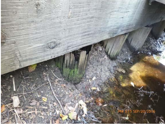
Figure 4.4 West abutment - Piles with major section loss.
