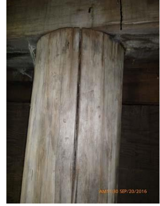
Figure 3.5 East abutment - Most piles are splitting and have internal decay.
