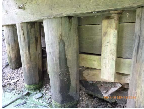
Figure 16.4 East abutment - failed backing planks and patches.
