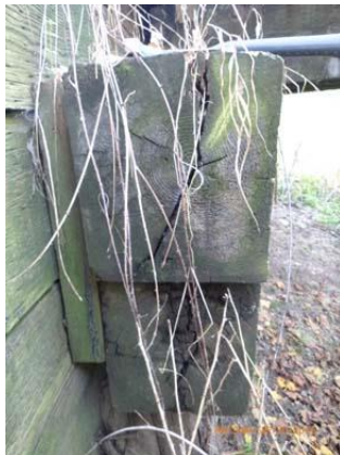
Figure 1.4 East Abutment - Splitting and rotating cap with 2x4 inch insert.
