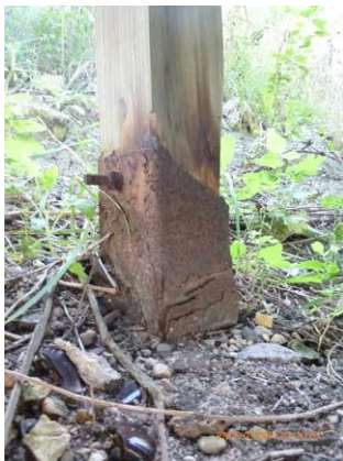
Figure 19.3 Footing brackets - Several footing brackets have active corrosion and section loss.
