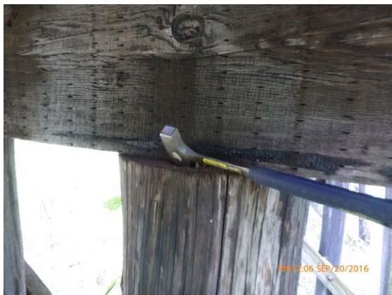
Figure 2.4 Pier 1 - Pile rotting and becoming hollow.
