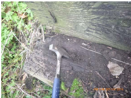
Figure 8.3 Footings - Section loss at the top on all corners.
