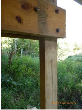
Figure 19.4 Pier posts - Minor splitting on some pier posts.
