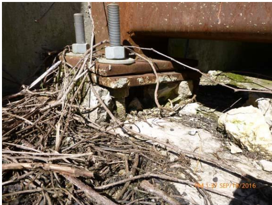
Figure 11.1 Southwest bearing - Bent anchor rods and spalled grout.
