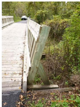
Figure 15.2 Rail - Failed floor beam supporting rail and kicker allowing for railing deflection.
