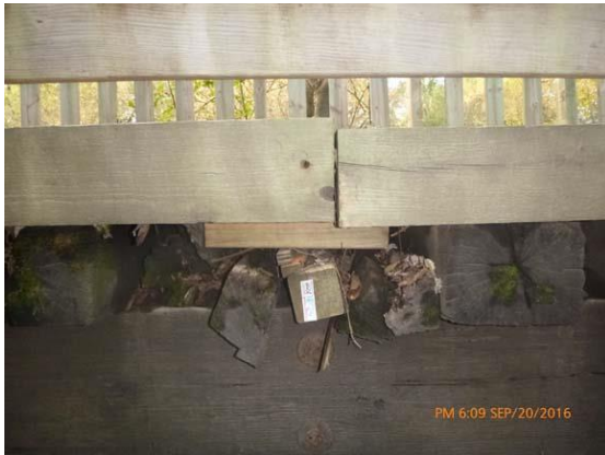
Figure 14.1 Floor Beam - Failed floor beam and patch.
