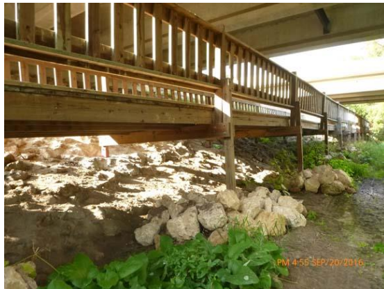
Figure 19.2 Piers - Riprap placed at the base of the posts holding well.
