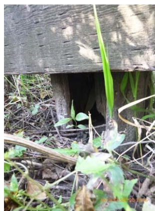
Figure 1.12 Pier 8 - Severe section loss inside the south pile.
