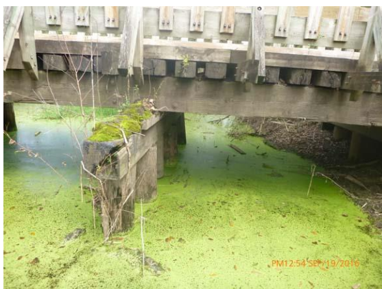
Figure 5.5 Pier 4 - Rotting pier cap and pile. Note minor impact damage on both fascia stringers.
