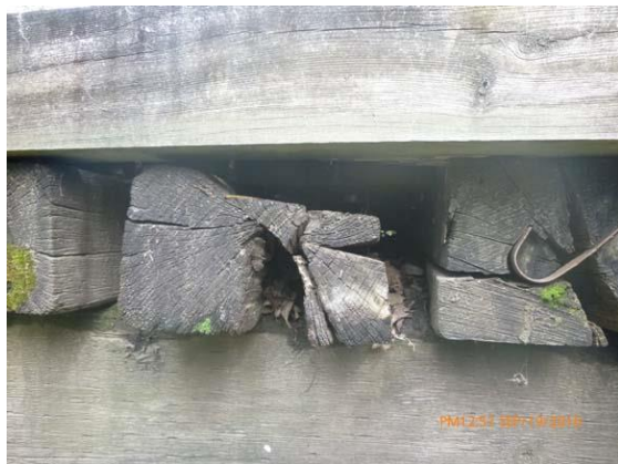
Figure 5.2 Floor beams - Failed floor beams throughout.
