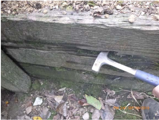
Figure 8.4 Footings - Section loss at the front on all corners.
