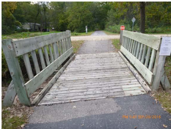
Figure 7.1 Deck - Bituminous and deck patches. Note how the southeast corner is slightly lower.
