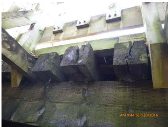
Figure 1.1 Floor Beams - Splitting and failing floor beams throughout the structure.
