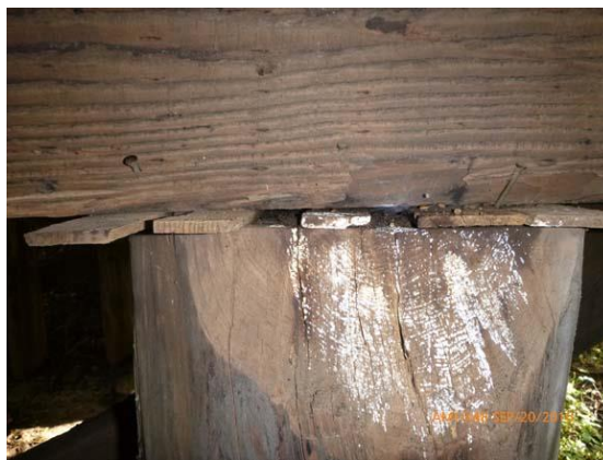
Figure 12.8 Piles - Rotting shims between piles and cap.
