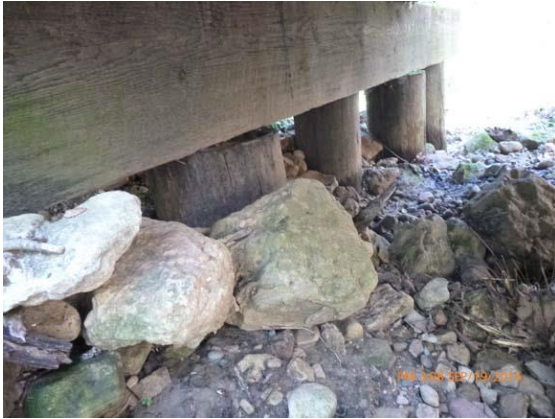
Figure 6.4 Pier - Piles becoming hollow.
