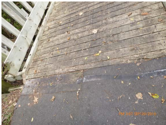
Figure 4.1 Approach - Wood plank used to patch bituminous approach.
