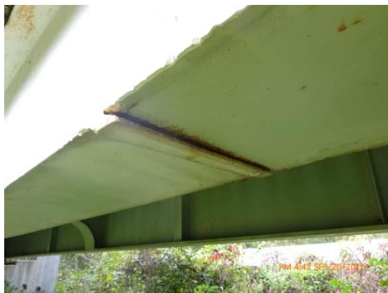
Figure 20.2 Beam - Construction joint separating.
