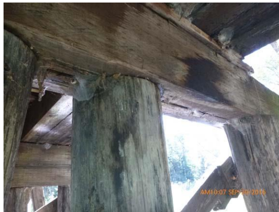
Figure 1.5 Pier 1 - Severe split running the entire length of the pier cap.
