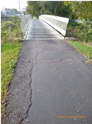
Figure 20.1 East approach - Extensive patching of the bituminous approach.
