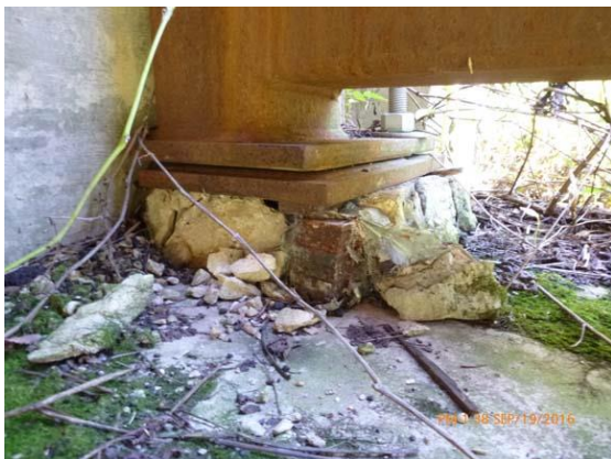
Figure 11.2 Northwest bearing - Bent anchor rods and spalled grout.
