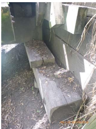
Figure 5.3 West abutment - decay and / or movement of bearing spacers, pile cap and backing planks.
