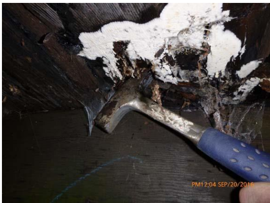
Figure 2.1 Beams - Section loss and rot at bearing area.
