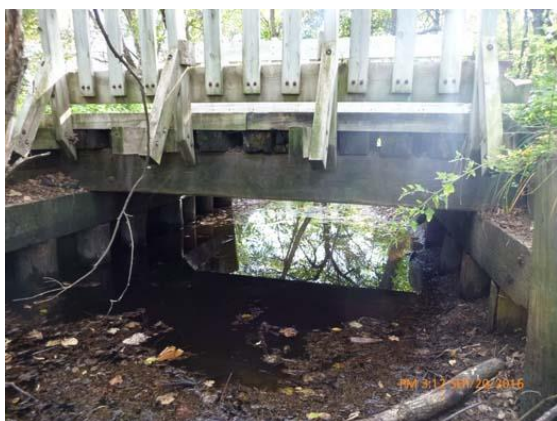
Figure 4.3 Abutments - Deteriorated and splitting piles.
