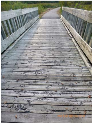
Figure 13.1 Deck - Moderate deterioration of the deck planks.
